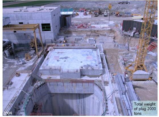
Fig. 11.8: The CMS plug after concreting
