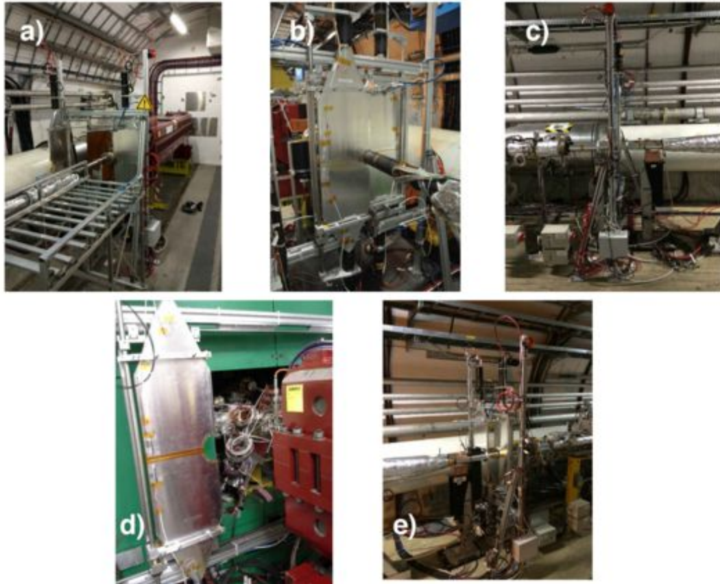
Fig. 9.4: Photographs of the installed Herschel scintillators in the LHC tunnel. a) shows station B0, 7.5 m upstream of LHCb, b) shows station B1 at 19.7m upstream and c) shows station B2 at 114 m upstream. On the downstream side, d) shows station F1, here in the open position such that the scintillator shape can be clearly seen, and e) shows station F2.
