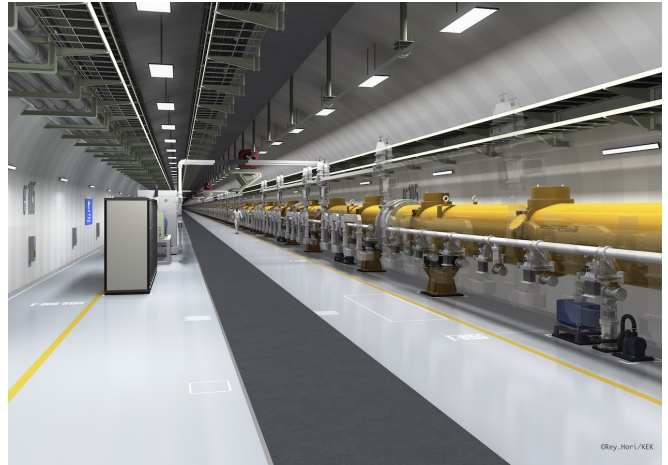
FIG. 12: Artist's rendition of the ILC Main Linac tunnel. The shield wall in the middle has been removed. ©Rey.Hori/KEK.
