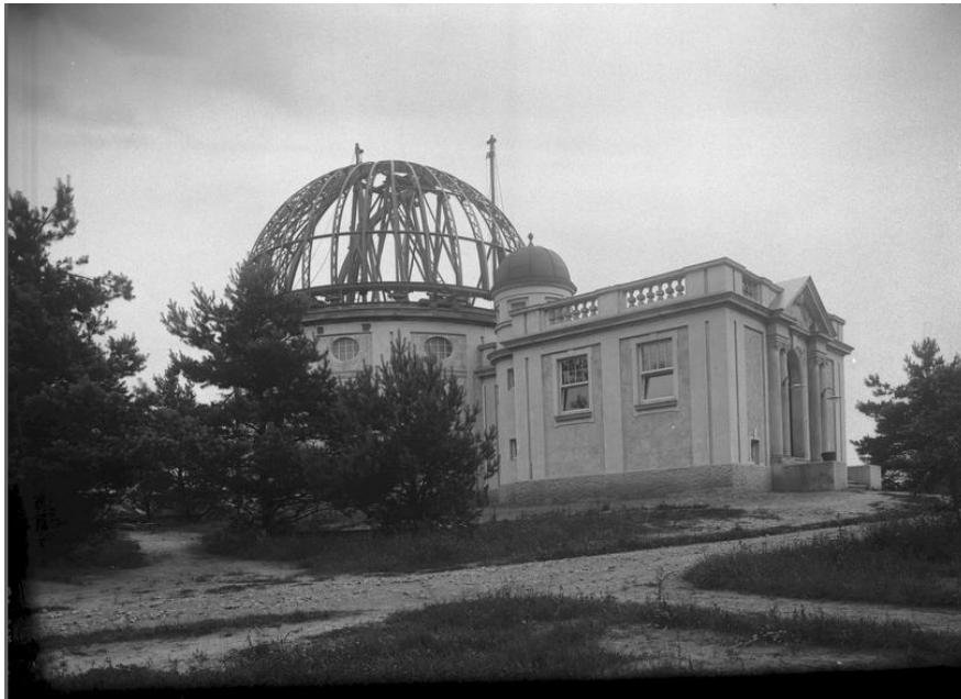
Figure 3: The dome housing the Great Refractor during construction. [1]
