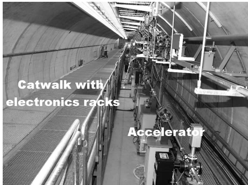
Figure 1: Tunnel of TESLA Test Facility II with crates for electronic systems in the catwalk
