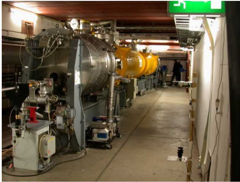
Figure 2.9: Inside TTF-2 tunnel, module 1.
