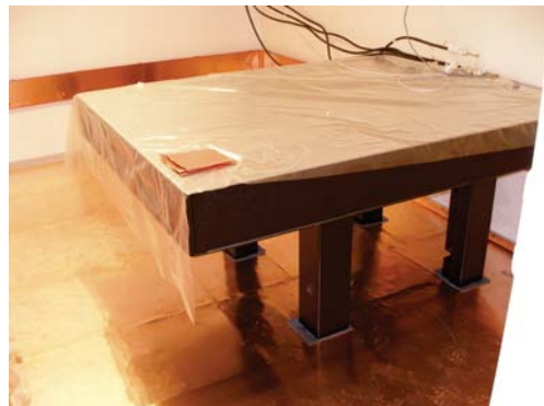
(d) Interior view during construction 3
