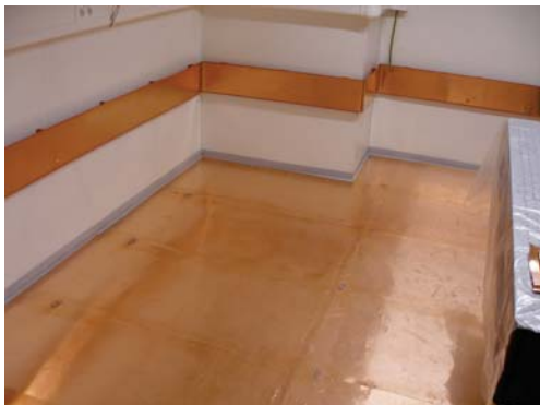
(c) Interior view during construction 2. The floor is covered with a 300 \mu\text{m} thick copper sheet.
