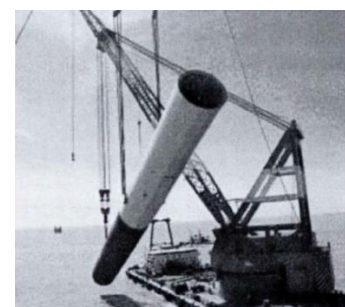
Figure 17. Construction of single-pile foundation [30]
