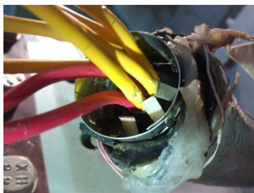
Figure 2: The damaged part of cable insulation
