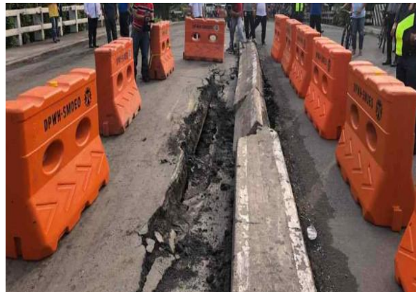
Figure 1. Cracks on Bridge Deck.
