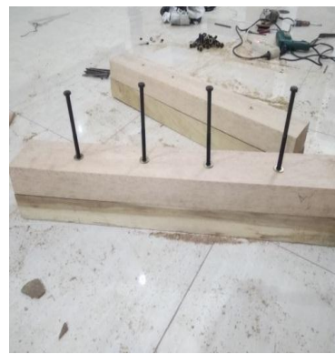
Figure 3. Bolt instalation
