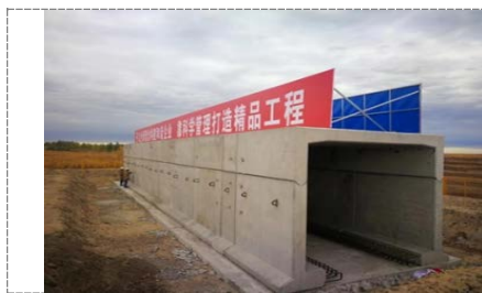
Figure 4. Box Culvert Roof and Side Wall Assembled Complete
