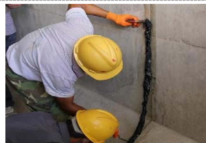
Figure 7. Construction of Asphalt Oakum
