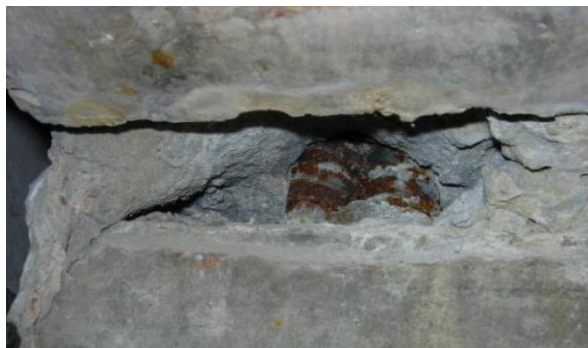
Figure 3. Non-concrete areas detected during the survey
