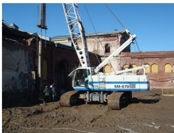
Figure 11. Construction of diaphragm wall during adaptation and restoration of Mikhailovskaya Dacha Building Complex to accommodate the Higher Police School Saint Petersburg State University campus
