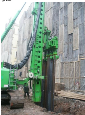
Figure 10. Indentation of the Arcelor sheet pile during construction of the basement of the business center at Nevsky Prospect, 55
