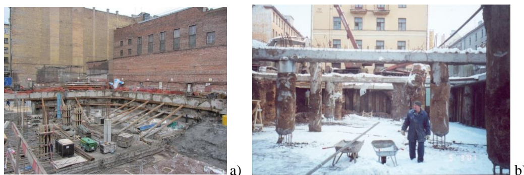
Figure 12. View of bracing structure in the form of struts (a) used in construction of Pravda-the Renaissance Office Center and reinforced concrete beams (b) on construction site of Business Center at Suvorovsky Pr. 2 (Semi-Top-Down construction technology)
