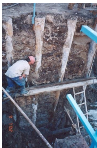
Figure 9. Construction of shoring of excavation pit using soil-cement mass when building pedestrian underpass in Avtovo
