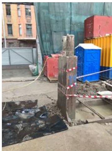
Figure 3. Installation of re-cage Figure 4. end stops: metal - extractable, reinforced concrete - lost.
