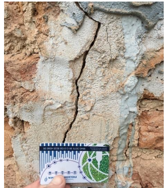
Figure 8. Diagrams of rise of deformation telltales and an example of opening of new crack at level of 2nd store.
