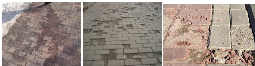
Figure 1. Fragments of the destruction of sidewalks made of concrete paving stones.
