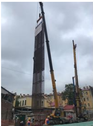
Figure 3. Installation of re-cage Figure 4. end stops: metal - extractable, reinforced concrete - lost.
