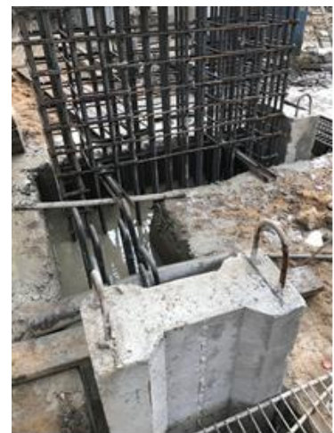
Figure 3. Installation of re-cage Figure 4. end stops: metal - extractable, reinforced concrete - lost.
