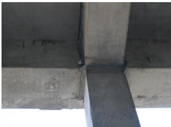
Figure 1. Crack opening in the pre-support zone
