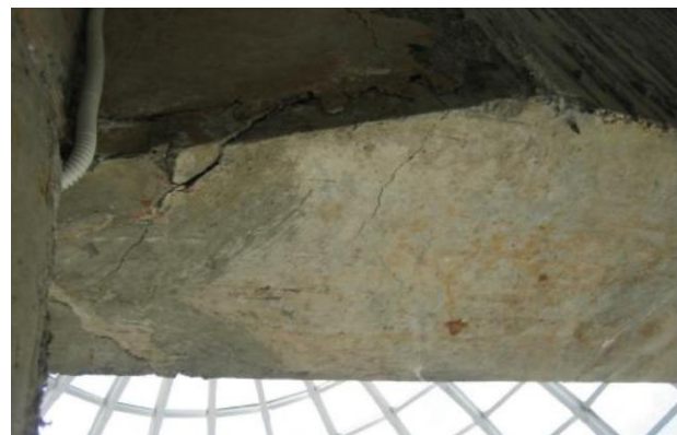
Figure 2. Opening of inclined cracks in the pre-support zone
