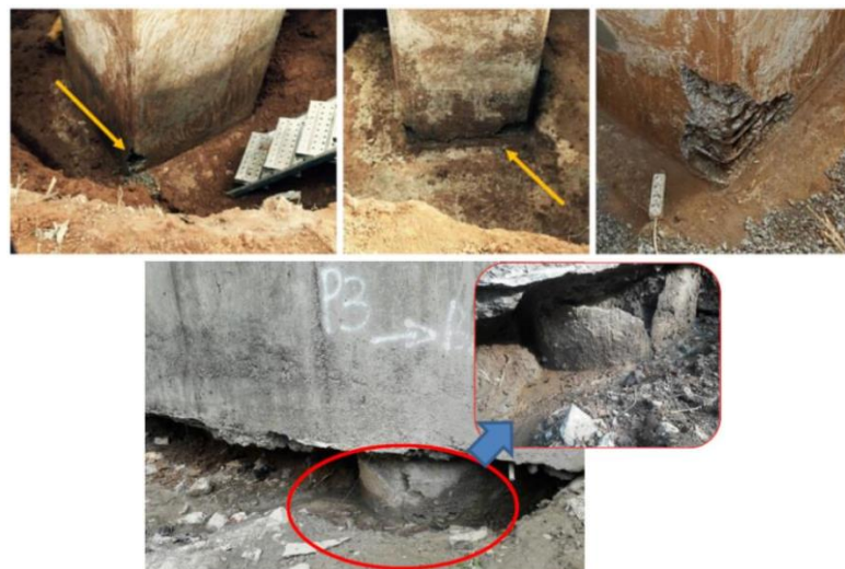
Figure 4. Structural damage on Cisomang bridge's piers [6].
