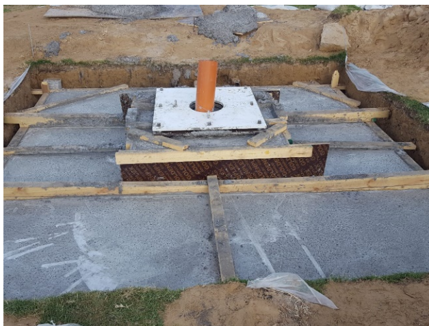
Figure 3. Foundation and mounting plate of the SPIDER 500A.
